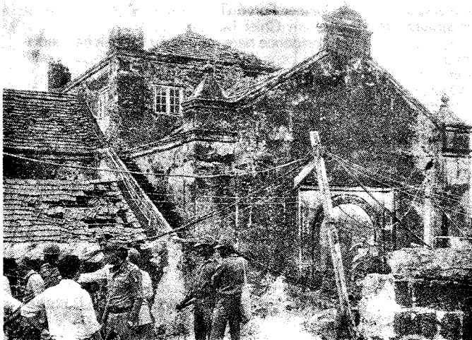
A historic landmark, the Jaffna Dutch Church built in 1706, damaged by shelling.
